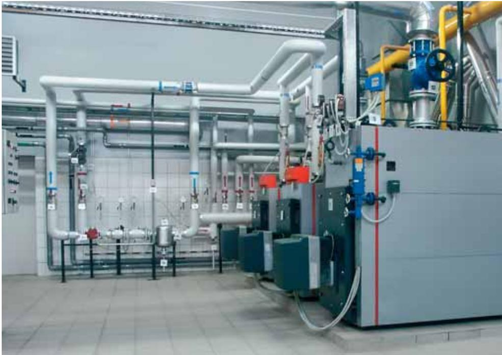
Typical application for smaller industrial premises: a Vitoplex LS (front) and two Vitocrossal boilers are in use here
