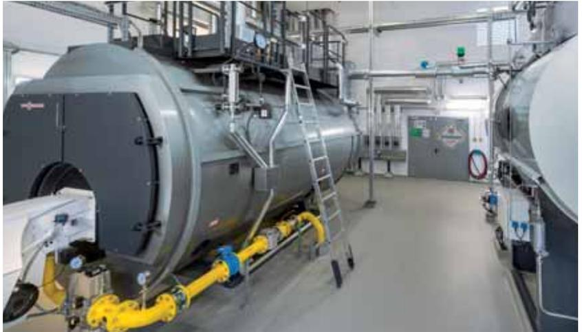
Vitamax HS with a steam output of 6 t/h and 10 bar pressure
