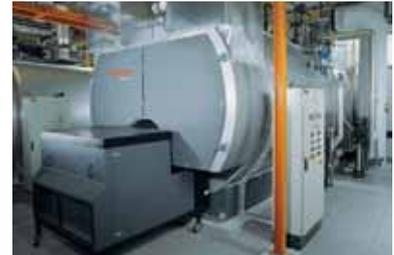
Vitomax RS steam boiler with waste heat utilisation and burner
