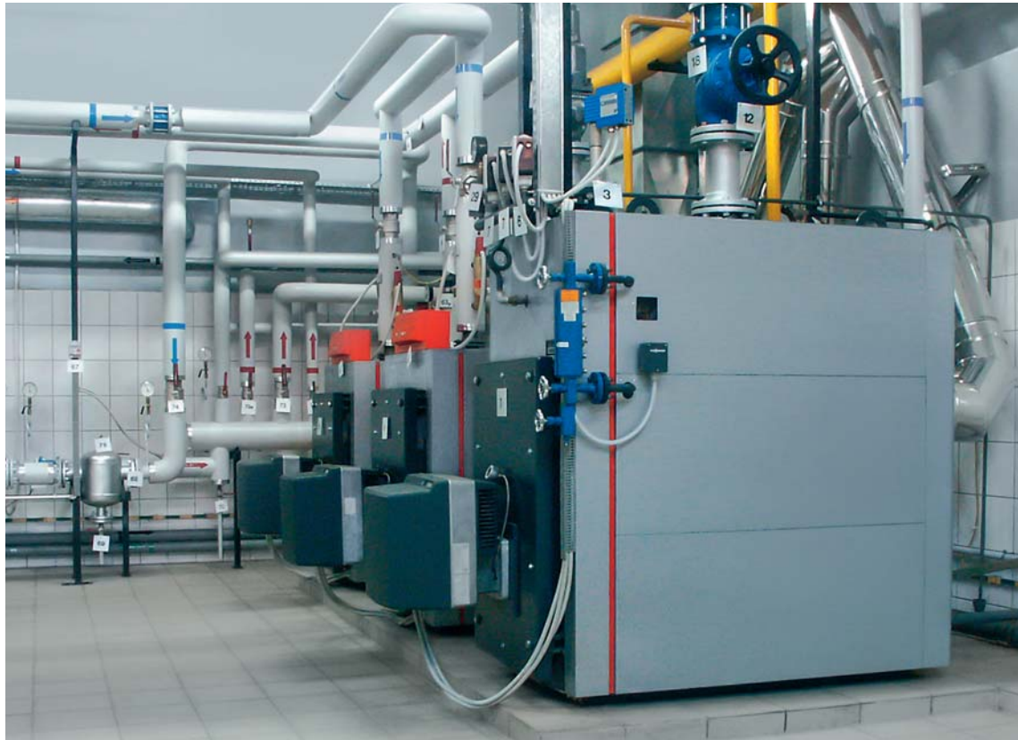
System with one Vitoplex LS low pressure steam boiler and two Vitoplex hot water boilers
