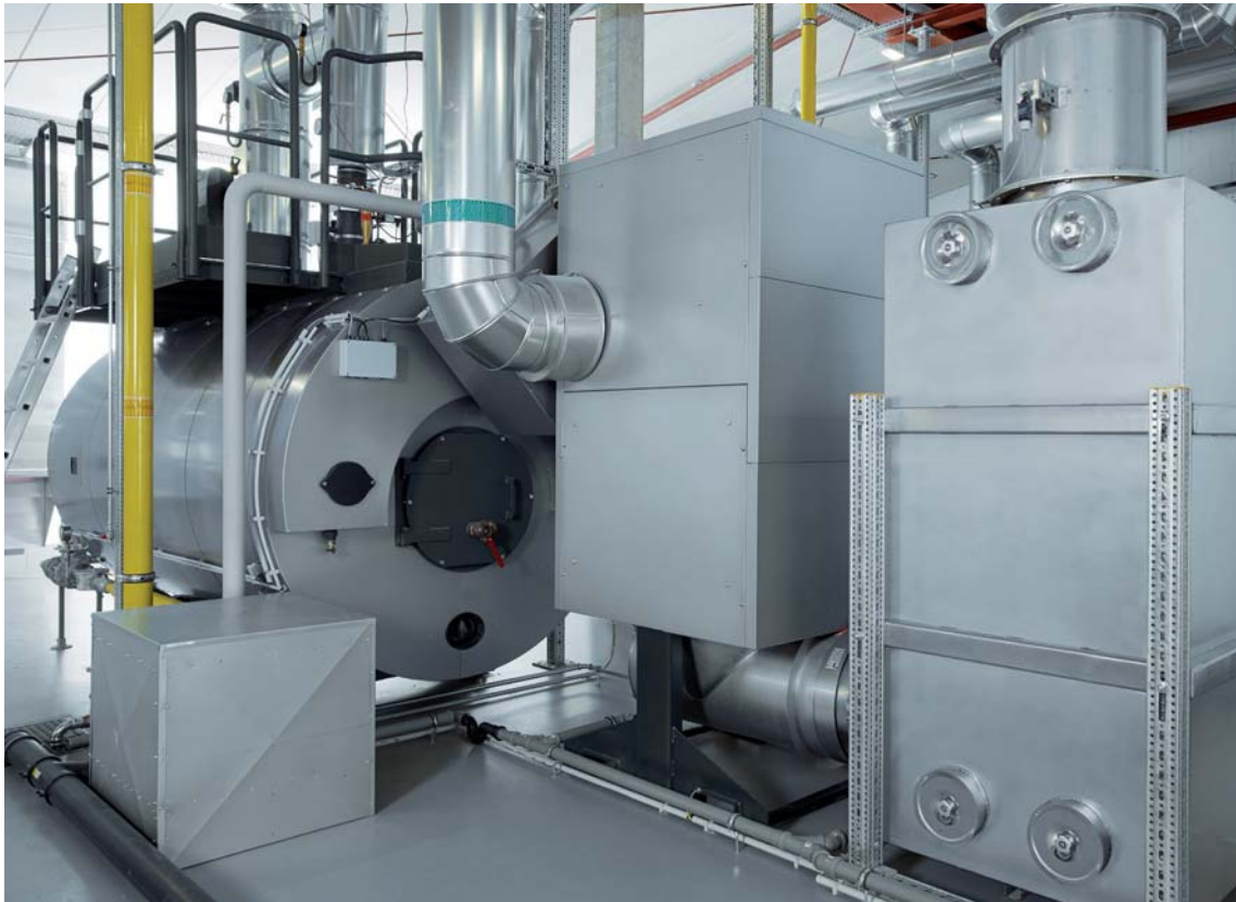
The Vitotrans 300 flue gas/water heat exchanger draws heat from the Vitomax boiler's hot flue gases and so improves efficiency.
