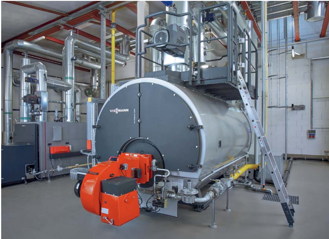
Vitomax LW hot water boiler (2300 kW) and Vitoplex 200 low temperature boiler (700 kW)
